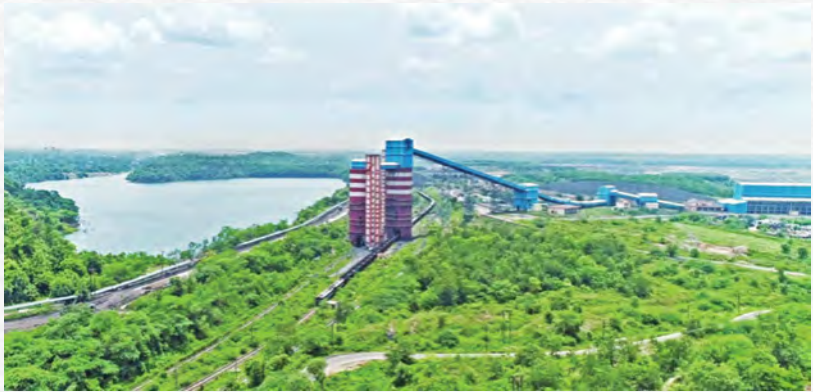
SILO AT BHARATPUR OCP
